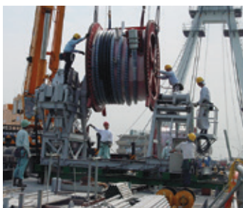
1 | Setting a cable reel on Unreeler
