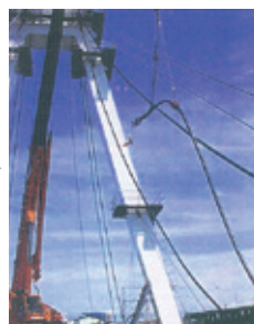
3 | Drawing & fixing of dead anchor
