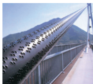
Indented cable: C_d \approx 0.7 ( C_d=0.7 is the same as smooth cable)
